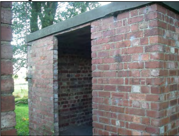
Photo 15: View of one of the disused RAF buildings
